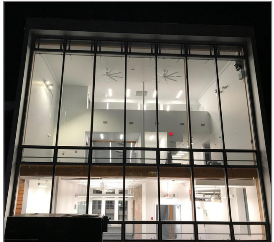
North facing rear façade
